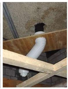
A pitch fibre connecting pipe from roof rainwater inlet into one of the long down pipes sealed in the corners of the upper brick walls below the lantern. Clear signs are visible that these have been leaking. Modern durable flexible plastic replacements were installed and sealed.
