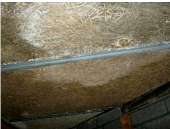
Because of the failure of the upper flat roof and leaking rainwater goods, clear signs of damp can be seen. Repairs to both have put a stop to this and damp areas have dried out.
