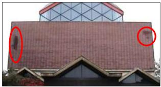
These views show (yellow) lower level leaks and (red) higher level leaks. At the lower level there seemed to be a regular height and regular interval, both inside and out, to the leaks. But what was inside the walls that could be leaking into the brick?
