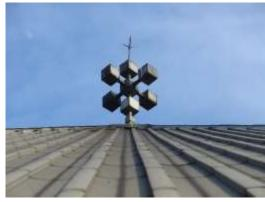
From ground level we had thought that the high level lantern fascia had faded paintwork but close inspection showed decay, as can be seen. All of this was renewed and the 'signature' 'bull's blood' colour of the porch lettering (and possibly, originally the foundation stone?) refreshed at this level, as had been originally when the church was built.
