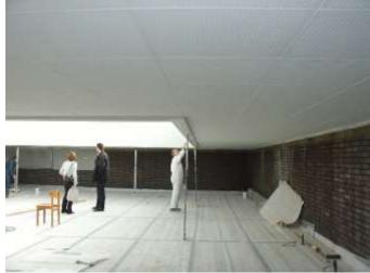
As the ceiling tiles were removed it was clear that there had been years of damp caused by water penetration though the failed upper flat roof asphalt and though leaking pitch fibre rainwater goods at that level.
