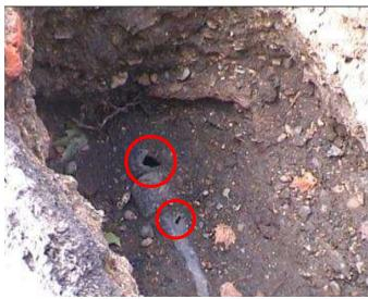
small section the pitch fibre had been perforated and almost certainly deformed or damaged elsewhere over a period which now well exceeds its useful maximum lifetime of 40 years or so.
