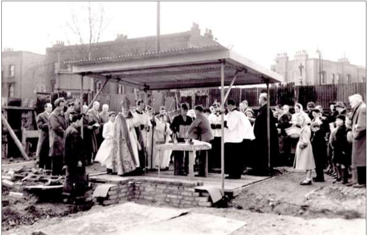
The Foundation Stone is moved into place
