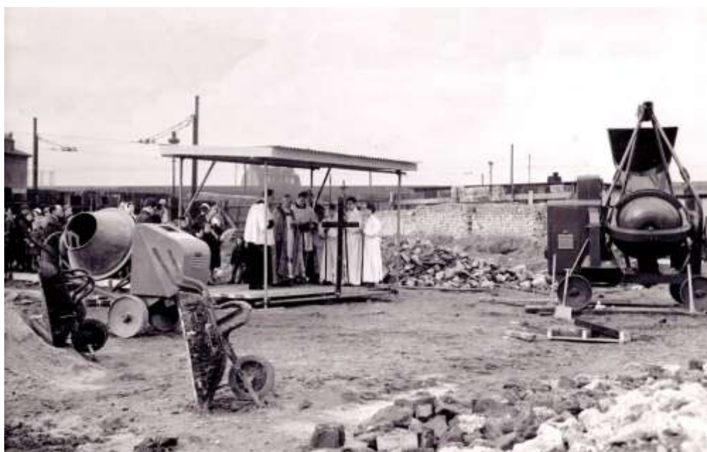
The building site
